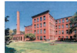
Robinson Cuticura Apartments Malden, MA
