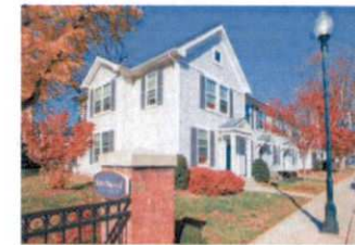
Southwood Square, Stamford CT 2017 RAD Conversion
